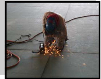
Leevac Shipyard employee Devin welds the first arc.
