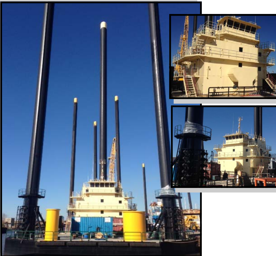
The M/V RAM XVIII currently under construction. Photos courtesy of Jude Bodin.
