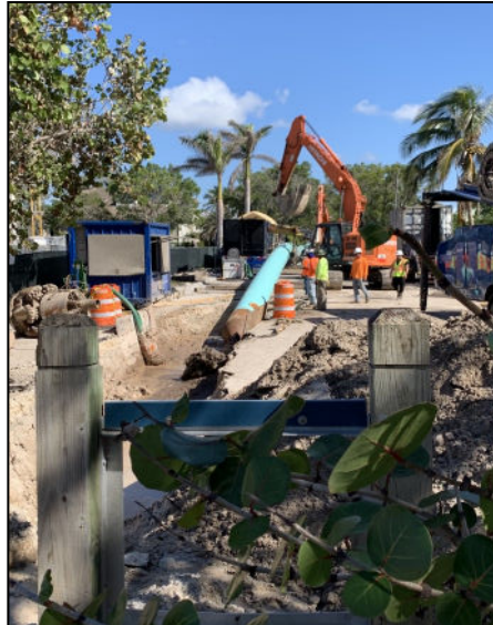
Dual 30-inch stormwater outfall pipelines
